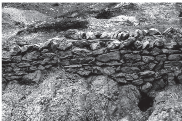
Sl. 2.17: Stavba 1, zid 3 – notranje lice. Detajl osrednjega dela zidu. Fig. 2.17: Building 1, wall 3 - interior. Detail of the central part.
