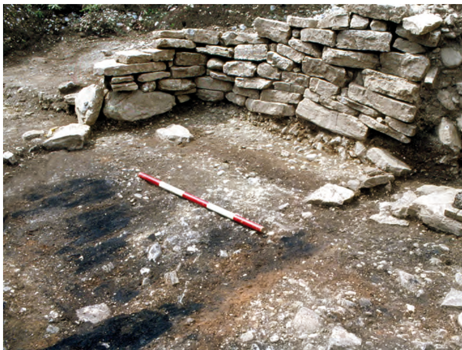
Sl. 92: Hiša 11. Vogalne plošče in ostanke zogljenega poda v zahodni polovici preddverja; pogled z vzhoda. Fig. 92: House 11. Corner slabs and charred remains of the floor in the west part of the entrance area; view from the east.
